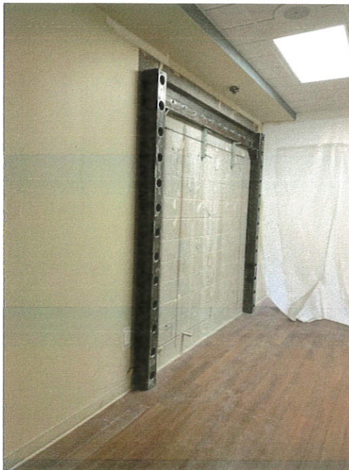
Photo of Steel Structural Supports
